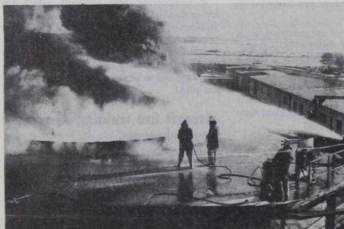
Using monitors to extinguish a large helideck fire
