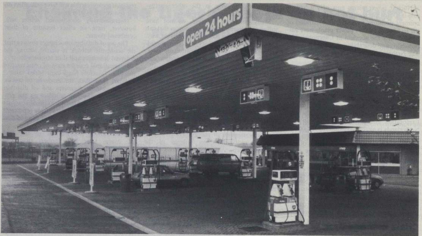
The largest service station in Europe, the BP South Mimms, on the M25, has multi product dispensers.
