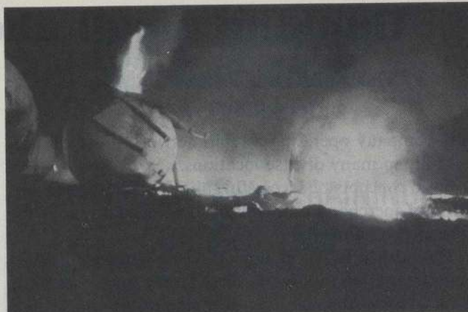
Storage spheres enveloped in flame in the Feyzin disaster. The conflagration at the Feyzin Refinery, France, caused initially by an operating error, took 48 hours to bring under control.
