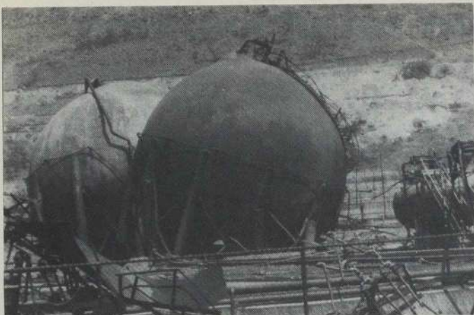
Two storage tanks left unexploded in the Mexico City disaster. Firemen may have prevented further explosions, but the extensive damage caused by the intense heat of the fire can clearly be seen.
