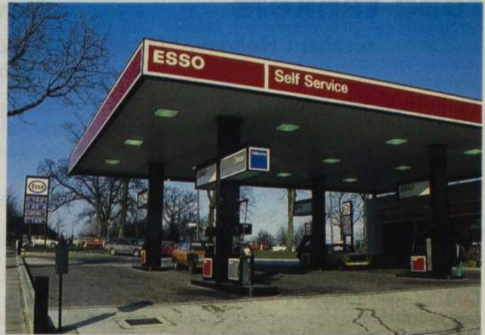
Esso's tigerish approach to station maintenance reinforces their commitment to Health and Safety, as well as good looks.
