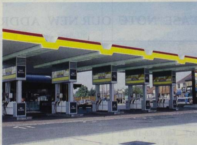
Shell: under canopy lighting, housed within heat bent and shaped opal diffusion panels, designed to enhance the unique canopy fascia profile.
