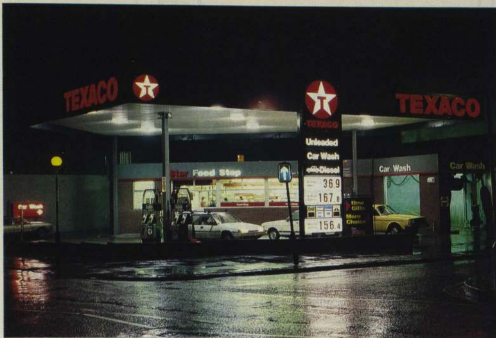
Texaco: dramatic nighttime shot demonstrating the use of extruded acrylic for the canopy fascia, graphics and logo.
