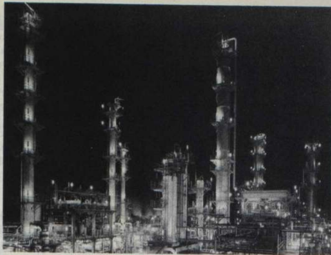
The unleaded petrol units at Lindsey Oil Refinery, South Killingholme on South Humberside. LOR is a joint venture between Petrofina and Total Oil (GB) Ltd.
