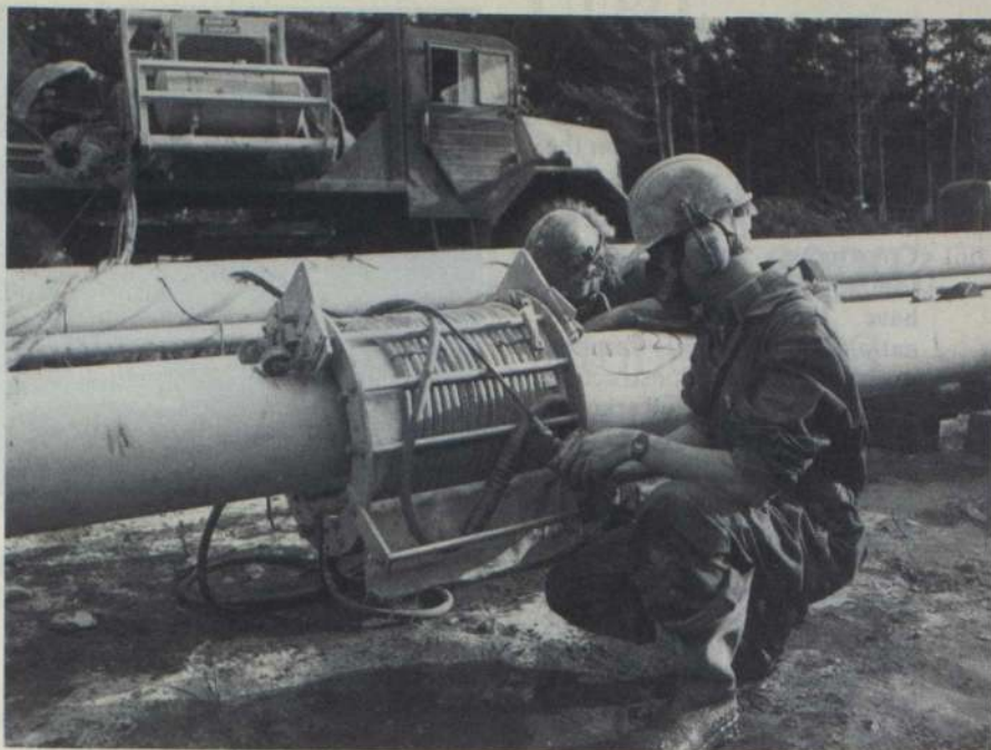
Epoxy coating of pipe joints on the Wytch Farm pipeline to BP Hamble Terminal on Southampton Water.
