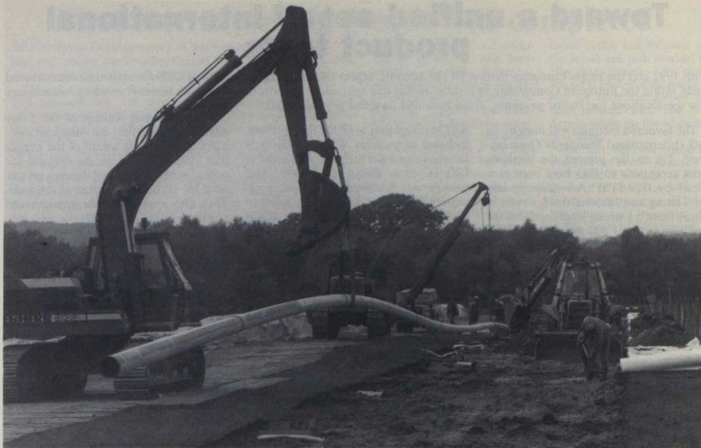
Pipe stringing on Creech Heath, one of the Sites of Special Scientific Interest on the Wytch Farm pipeline route.
