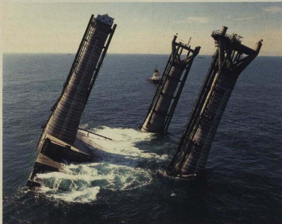
The concrete gravity structure during its successful inclined installation last month at the Ravenspurn North development, operated by Hamilton Brothers. Designed by Ove Arup and constructed by John Laing ETE Ltd, it is a shallow water version of the platforms described in this article.
