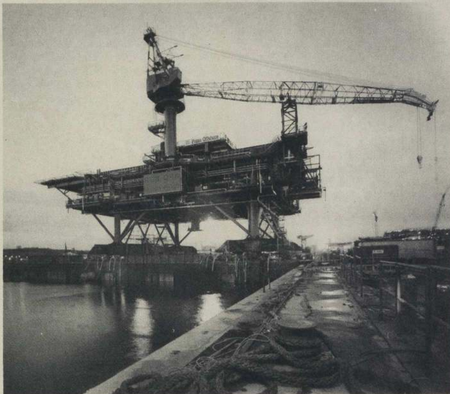
This integrated deck was built by Press Offshore for the Morecambe Bay gas field.
