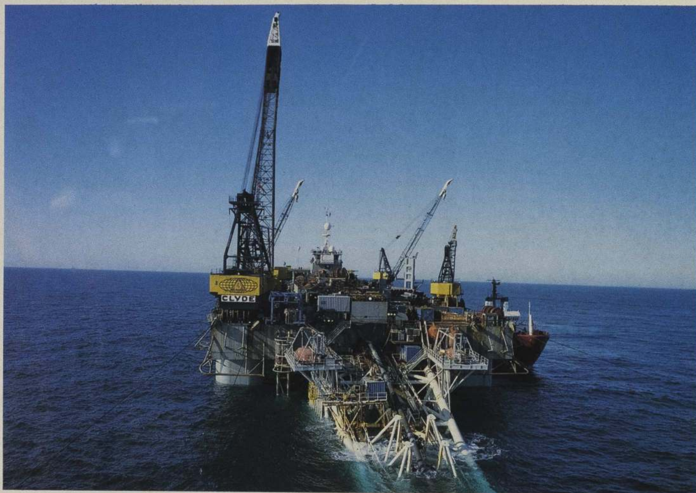
Pipelaying in the northern North Sea.
