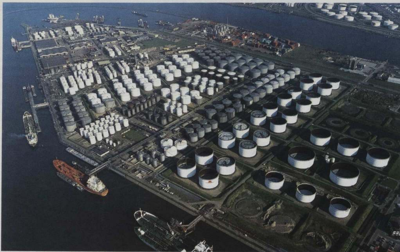
Paktank's Botlek Terminal.
