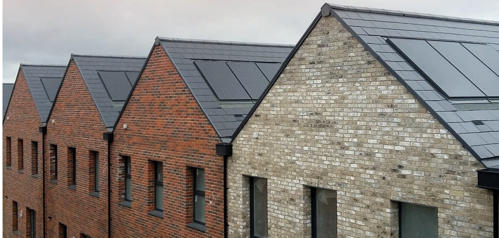
New homes featuring slate roof-integrated solar PV Photo: Viridian
