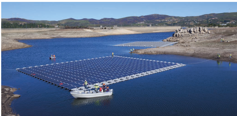
Floating photovoltaics at the Alto Rabagão pumped storage reservoir, Portugal Photo: EDP 3
