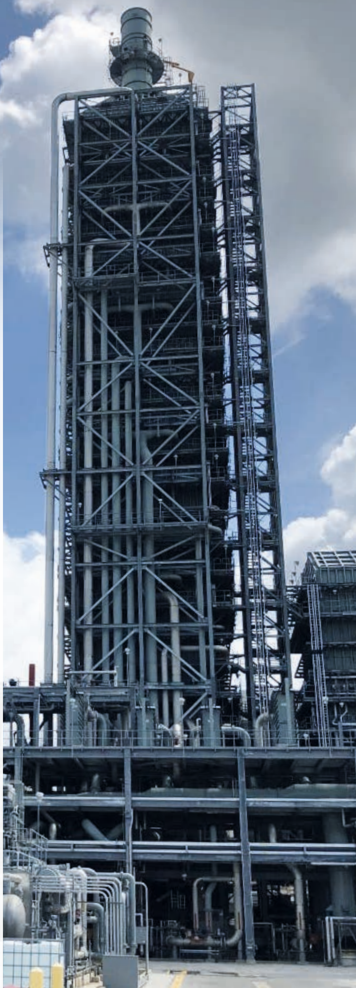
The Petra Nova CCS facility uses post-combustion CO 2 capture at a US power plant Photo: Global CCS Institute
